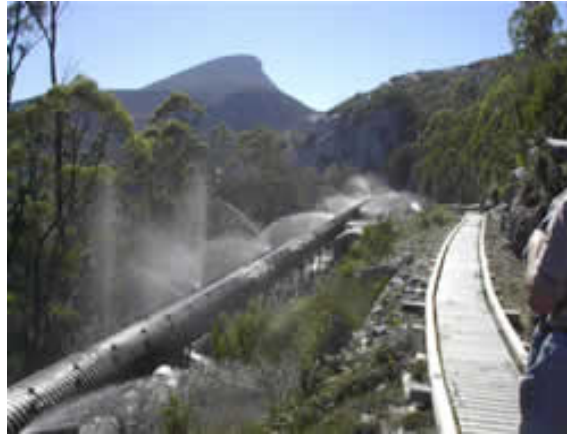
Pic 2: The old King Billy Pine Pipeline "Soaker Hose"
