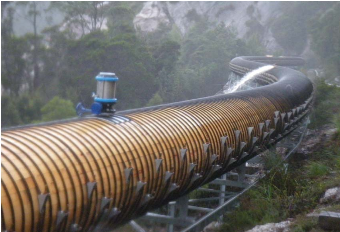
Pic 1: The new 1200mm Alaskan Yellow Cedar Woodstave Pipeline at Mt Margaret, Tasmania
