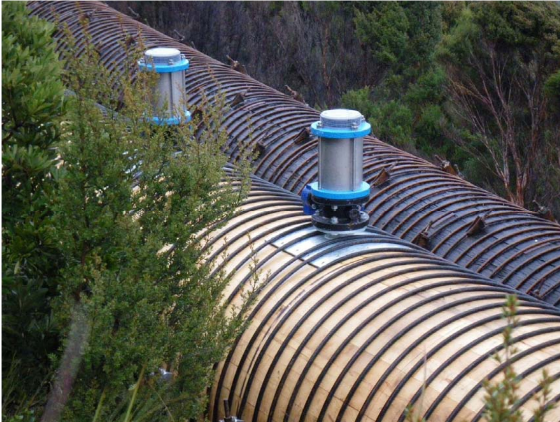
Pic 3: Old and New Pipeline side by side
