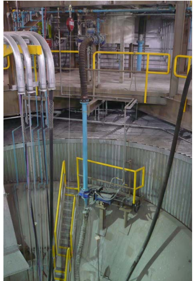
4" RF VALVE modulating w/digital control
